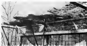
Figure 61. Netting garrisoned with steel wool distorts the shape of this building from aerial view.
